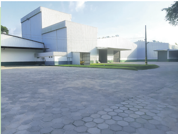
Paving of the areas surrounding the industrial facilities.
